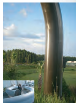
Florida State Piping Project U.S.A
