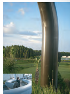
Florida State Piping Project U.S.A
