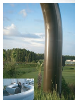
Florida State Piping Project U.S.A
